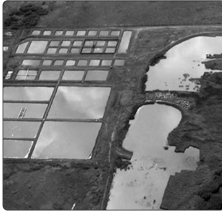
Figure 2.1-1. Ponds at the Moi University Fish Farm are neatly laid out, with water flowing by gravity from the water reservoir (right) to the ponds (left).
